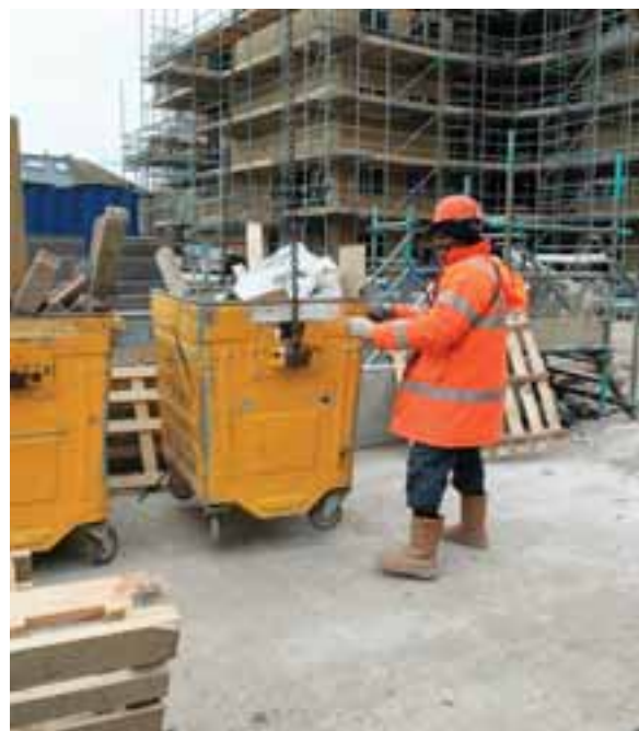
On-site separation of construction waste. Credit: WRAP
